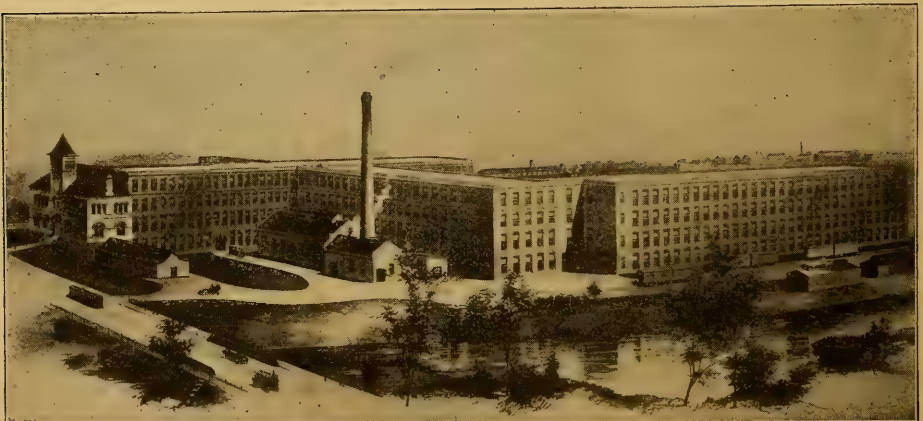
Plant of the Electric Vehicle Company, Hartford.
